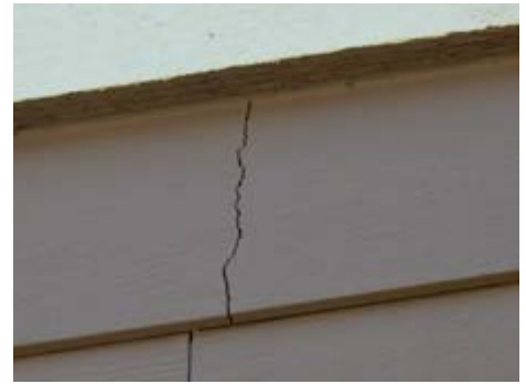
Siding cracking
