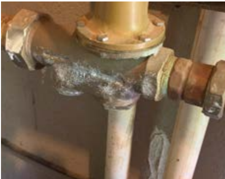
Fitting corrosion
